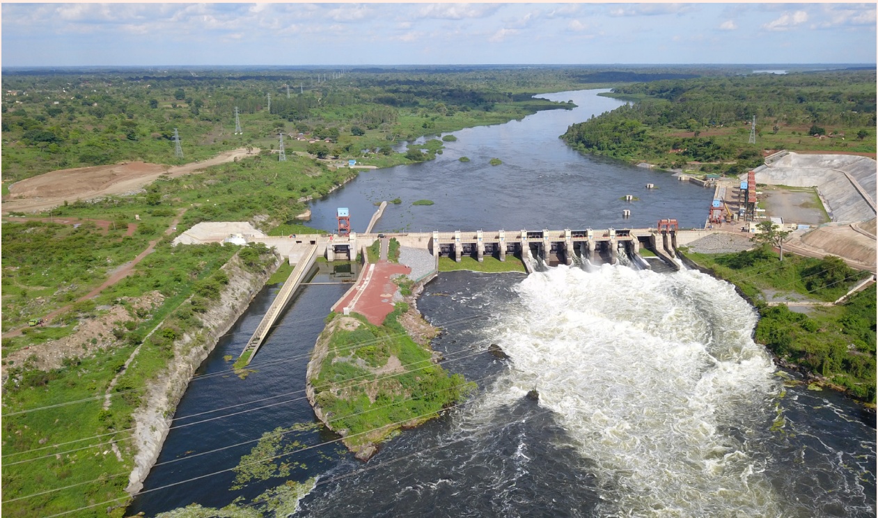
This photo taken on December 14, 2024 shows the Chinese-built Karuma Hydropower Plant in Kiryandongo, Uganda. Uganda on February 6, 2024 successfully launched the last unit of six turbines at the Chinese-built Karuma Hydropower Plant and synchronized it on the national grid, the country's electricity generation agency said. (XINHUA)
